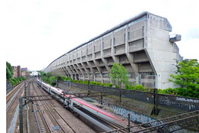
fig 189: The machine-like back of block A as a noise barrier
